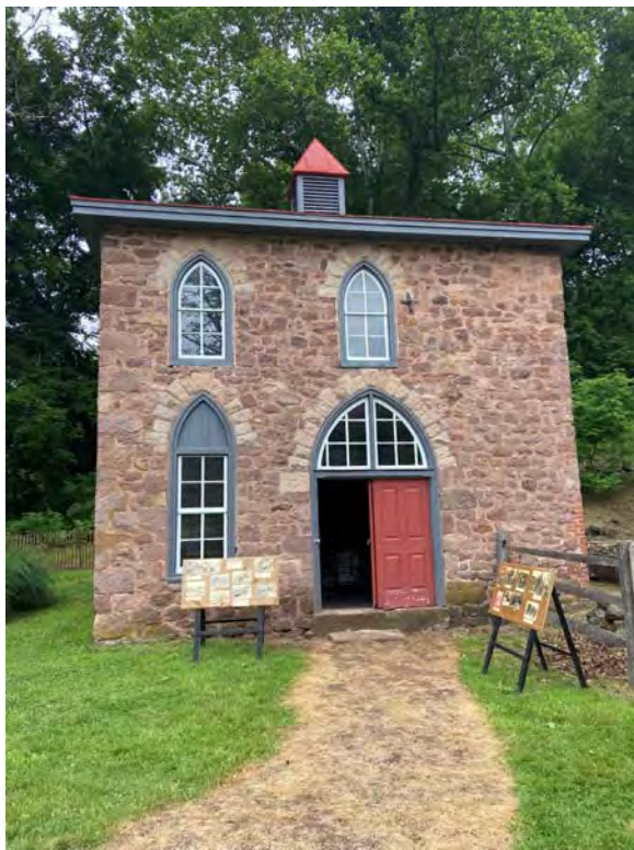
Blower Engine House, Joanna Furnace
