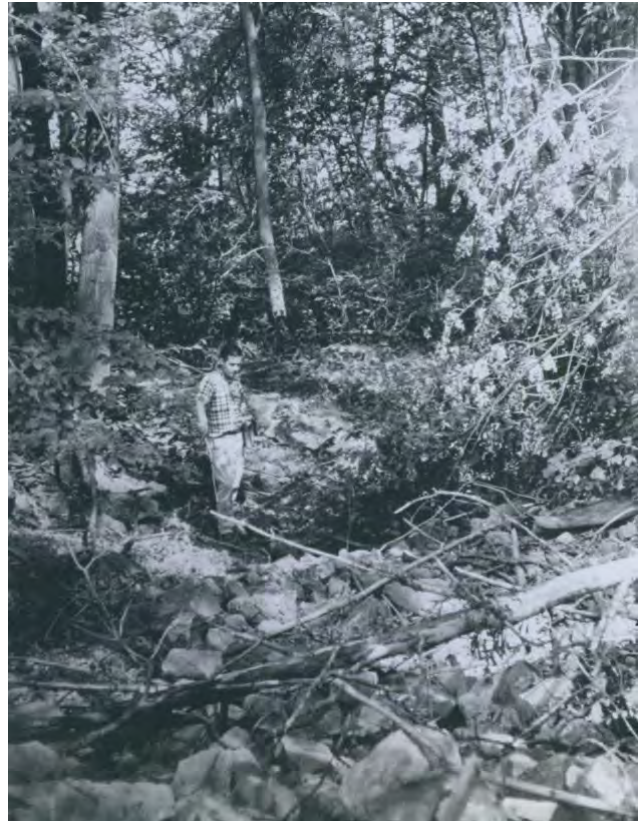
View of quarry depression at the Vera Cruz (36LH0012). Photo dated August 24, 1967
